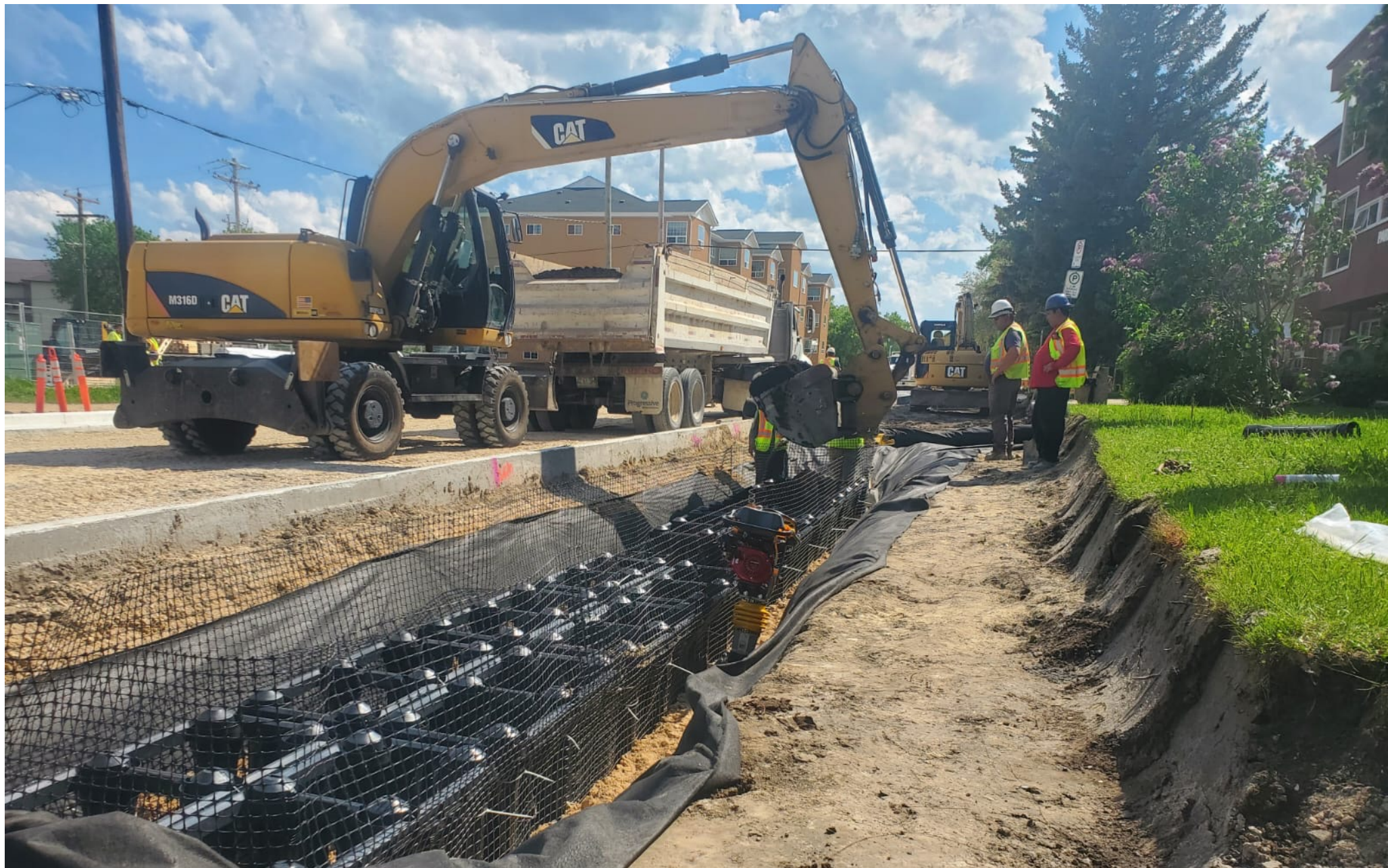
SILVA CELL INSTALLATION
